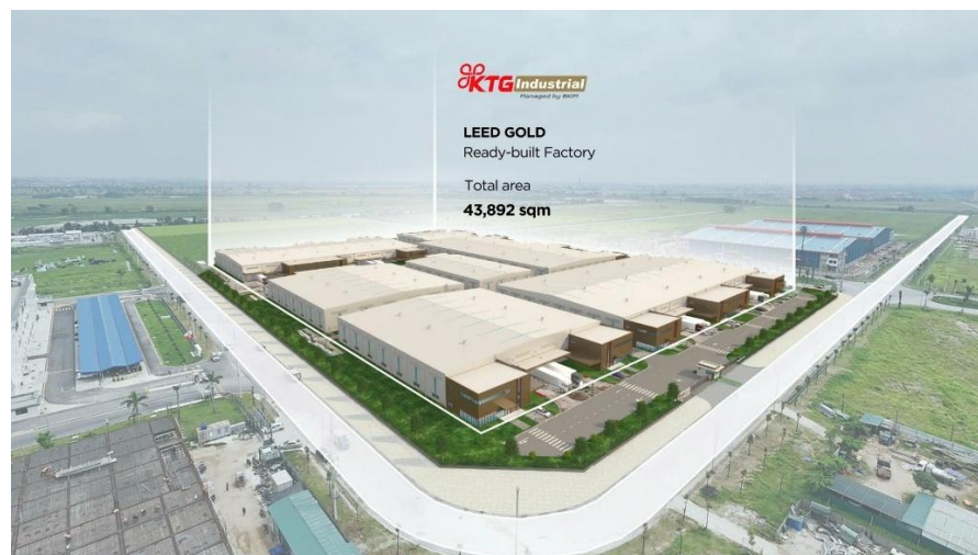
KTG Industrial VSIP Bac Ninh 2, 출처: KTG Industrial
