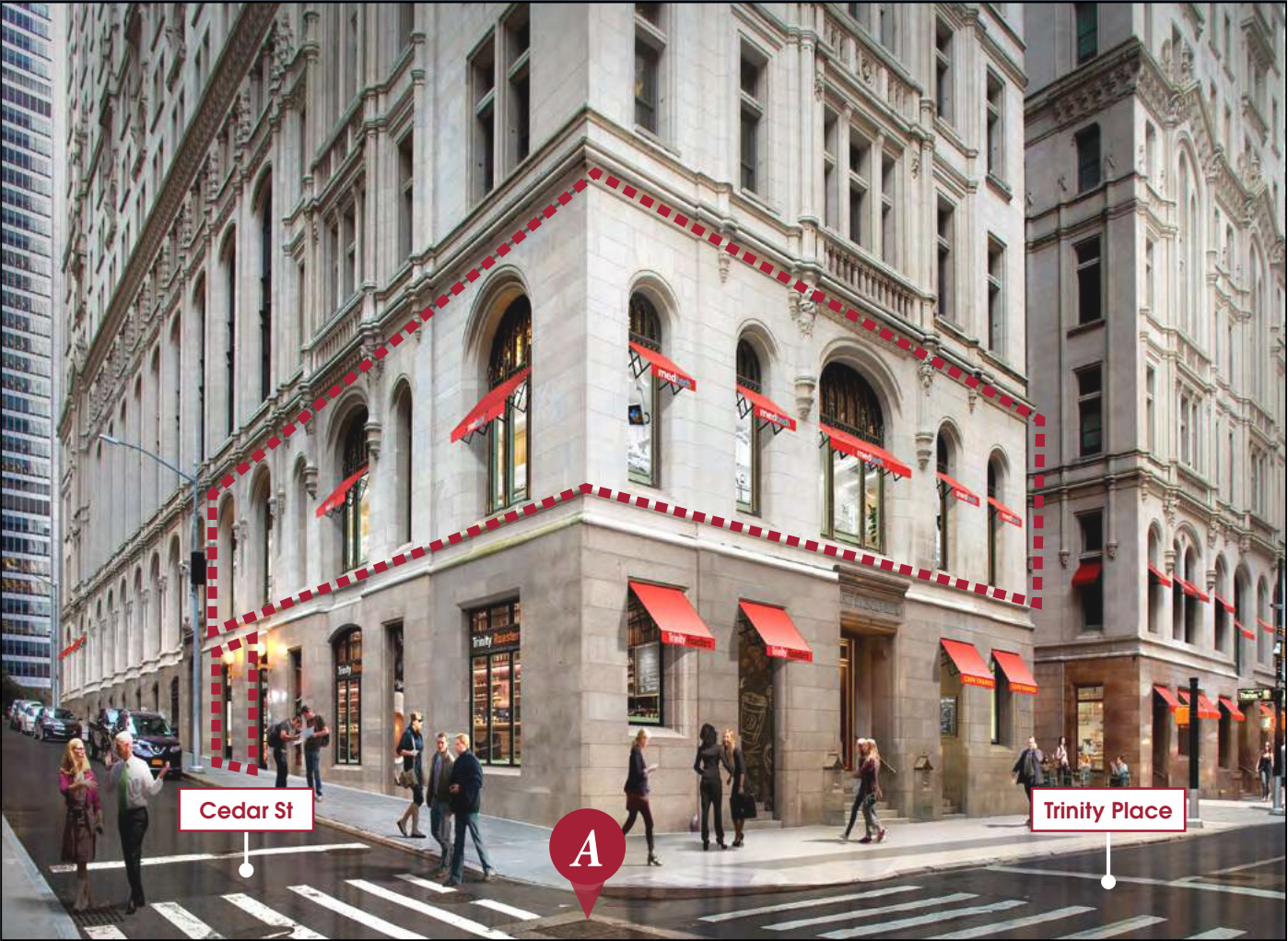
2. Cedar Street and Trinity Place frontage and access
