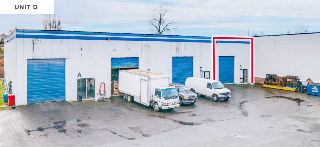
UNIT D WAREHOUSE
