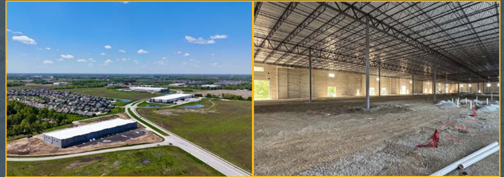
STEEL AND ROOF COMPLETED
