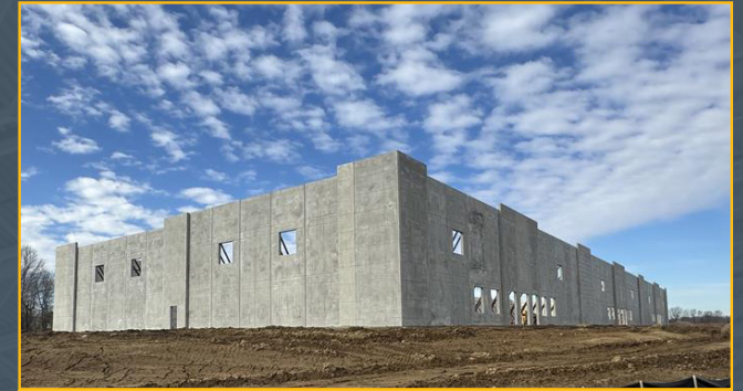
WALLS GOING VERTICAL
