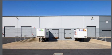
Grade Level and Dock Height Loading Doors
