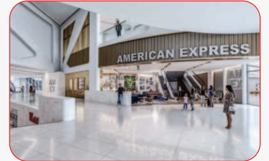
Future Amex Lobby
