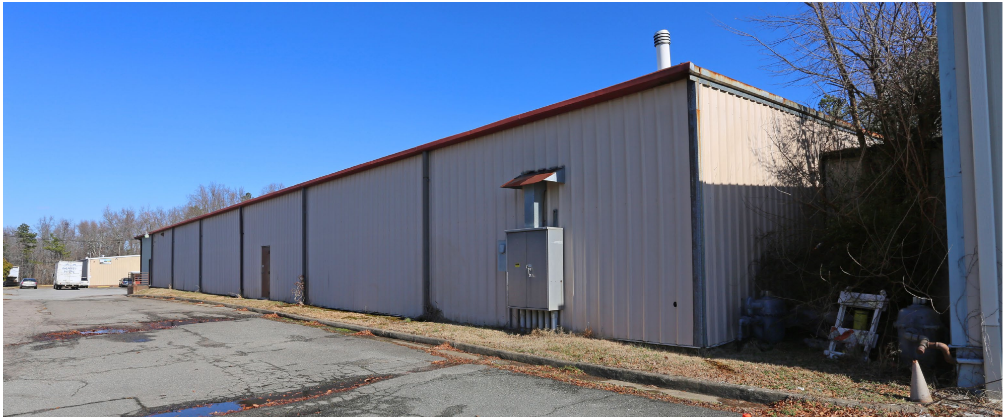
REAR OF THE BUILDING
