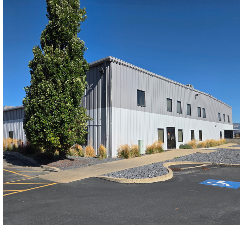
Building 3 | 23,508 SF Available
